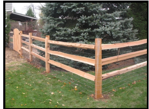
Split Rail with Wire
